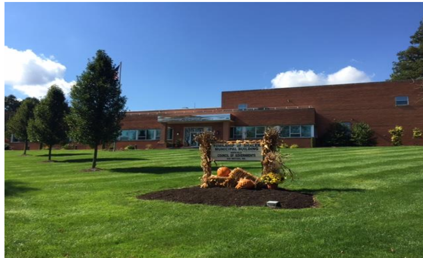
SHALER TOWNSHIP MUNICIPAL BUILDING 300 WETZEL ROAD, GLENSHAW, PA 15116
