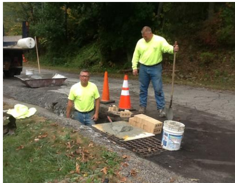
Replacement of Storm Sewer on Lehr Avenue
